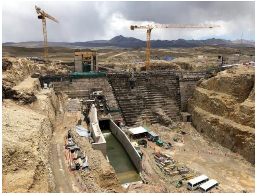
Figure 16: Vizcachas Dam lo- level outlet and stepped spillway
